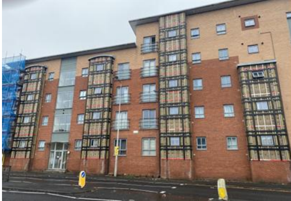
A photo showing Elevation Ready For Panels
