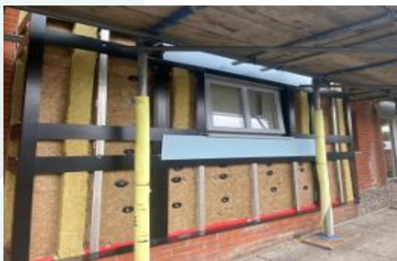
Photo Showing Progression On C1 Panel Install
